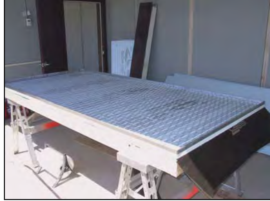
Figure 3. Foam sheathing test wall
