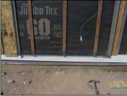
Figure 2. Strapping that creates ventilated cladding
